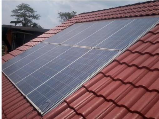
Figure 1: The PV installation on the roof
